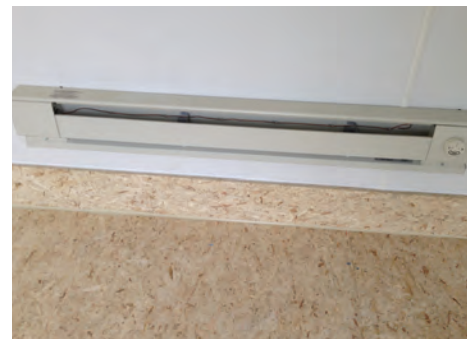
BASEBOARD HEATING SYSTEM - A must for the year-round roving workshop. The self-contained unit comes with an optional adjustable thermostat control.
