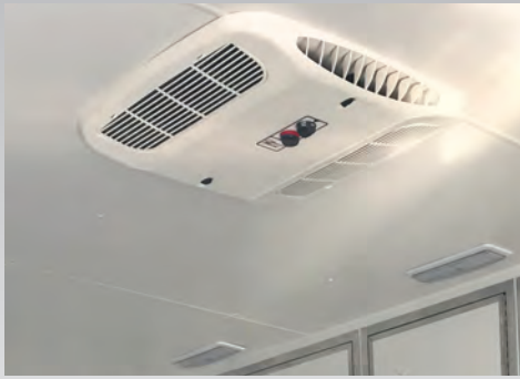
ROOF AIR CONDITIONING - This roof mounted air-conditioning unit has directional vents, variable temperature knob, and three-position cool and fan.
